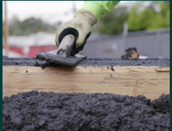
Spreading OurCarbon® enhanced concrete on footings
