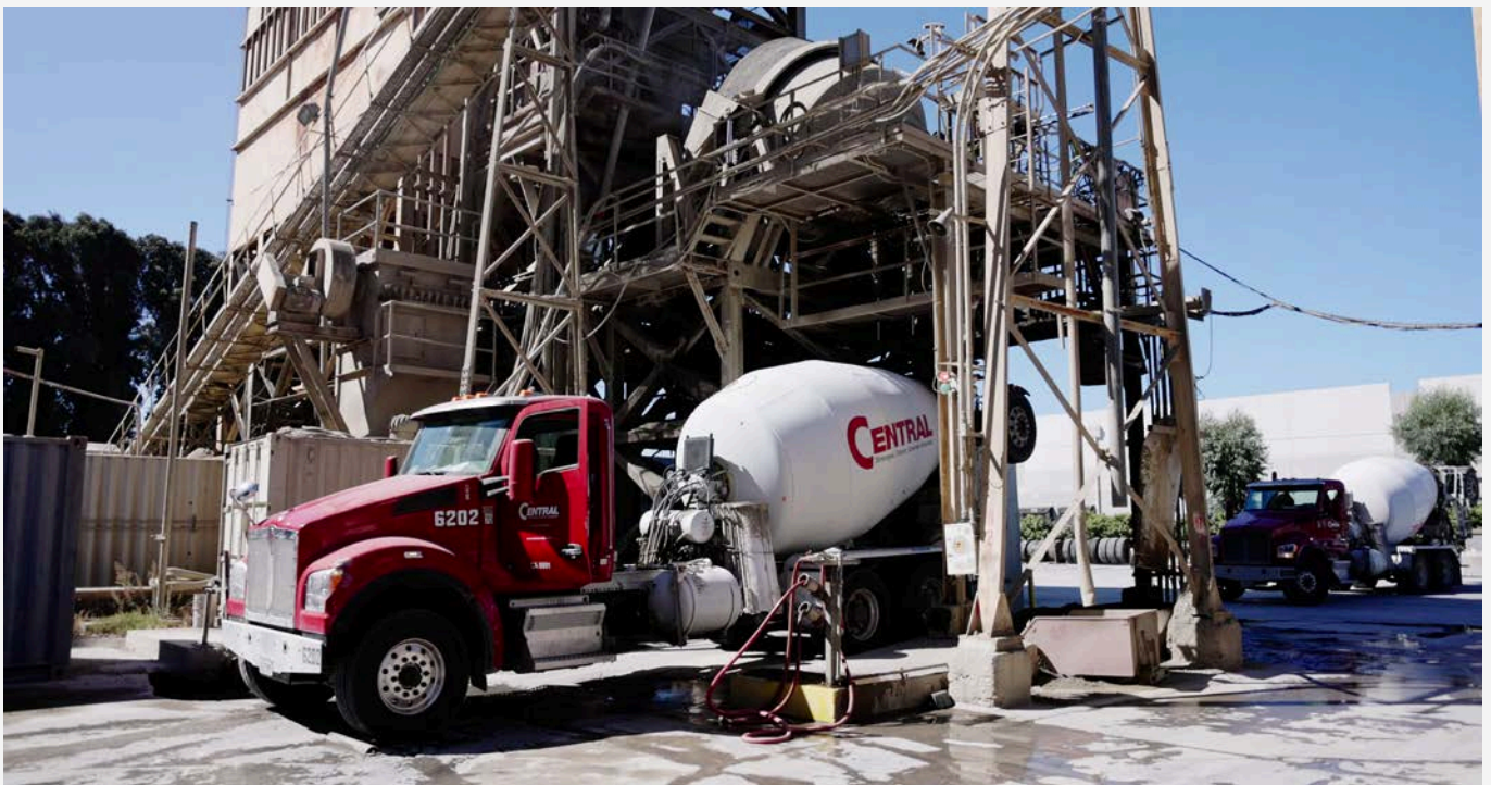
Central Concrete truck collecting mix material
