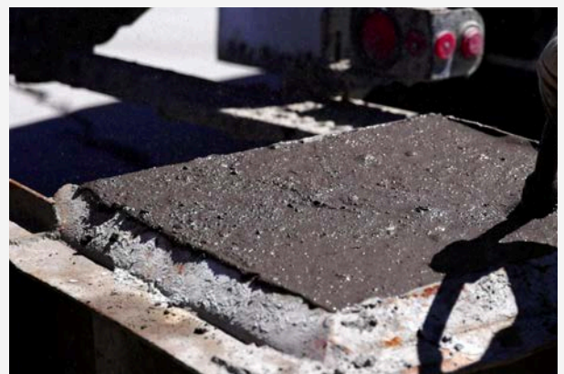
Final testing to ensure concrete workability
