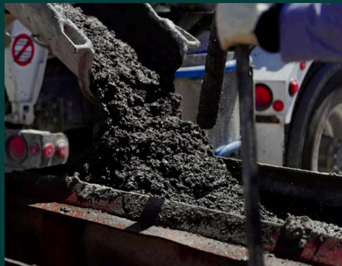
OurCarbon® enhanced concrete being poured by Central Concrete.
