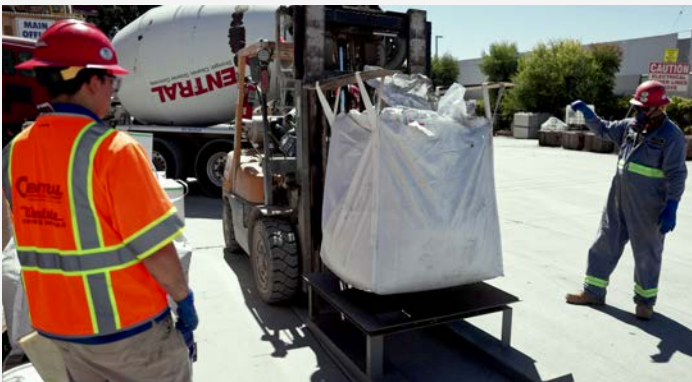
Mixing OurCarbon® with Central Concrete's mix
